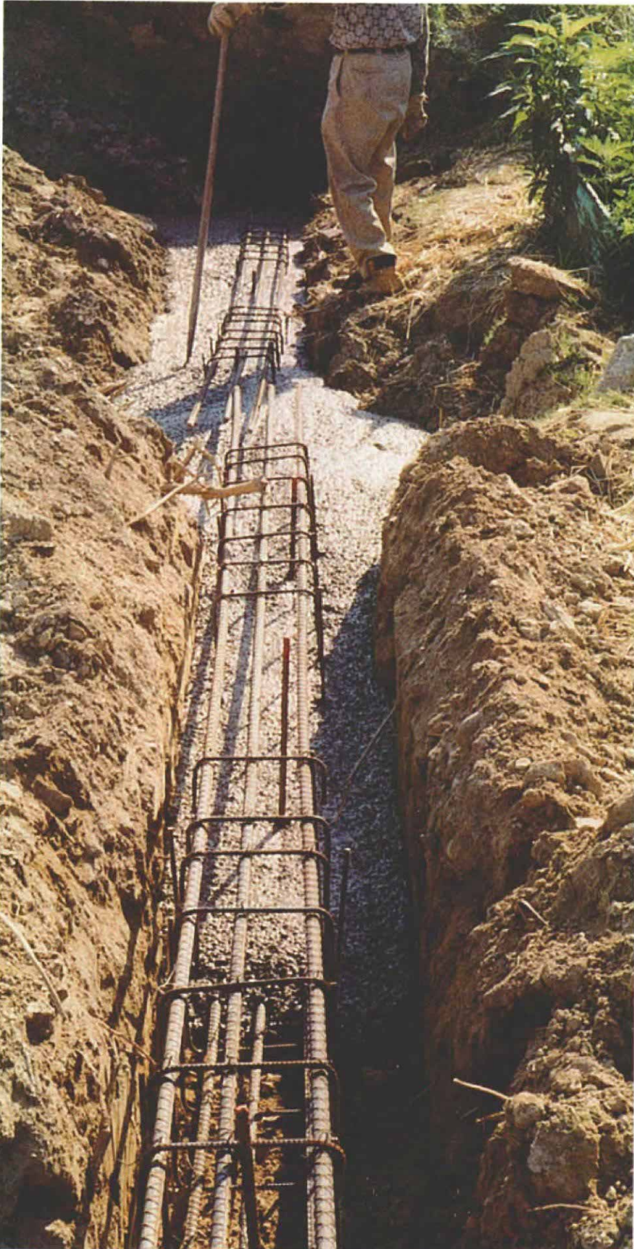
Adequate reinforcement. A grade beam must resist bending forces from any direction. Forming the rebar into a cage provides reinforcement across the beam's entire cross section.
